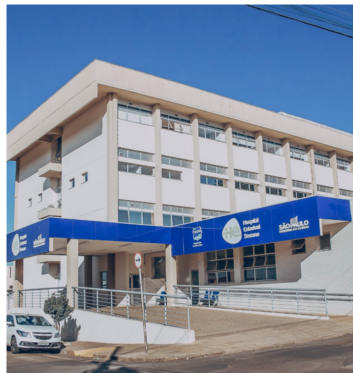
O Hospital Estadual de Serrana/SP.
